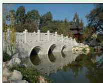
Jade Ribbon Bridge
