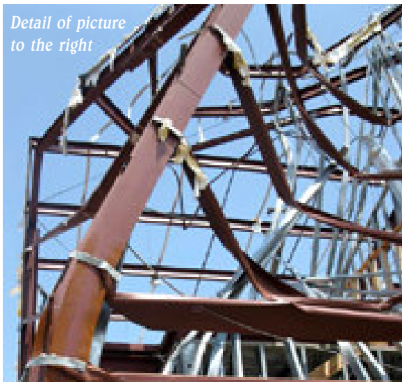
The tornado twisted the steel girders of this bank building under construction
